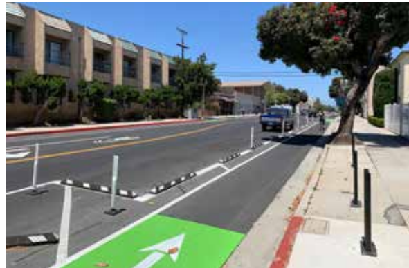
Flexible posts and striped buffer protection.
