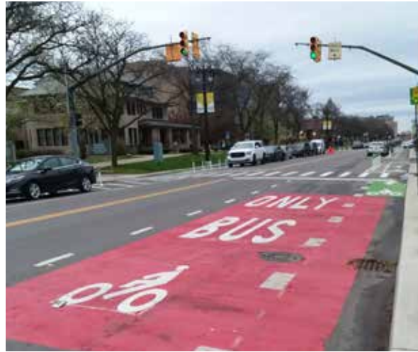
Bus/bike mixing zone at a bus stop on the Cass Avenue protected bikeway in Detroit. Source: Nelson\Nygaard
