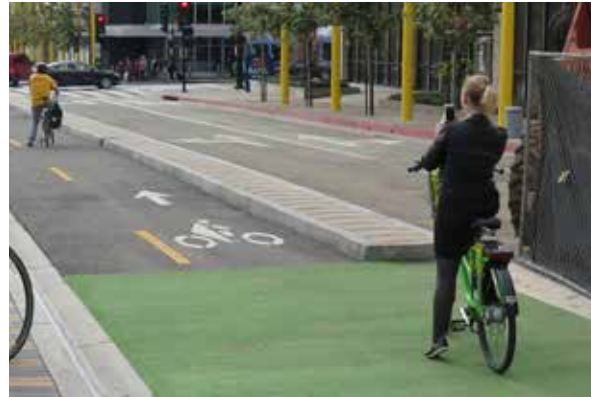
Raised curb protection on Colorado Ave Esplanade.
