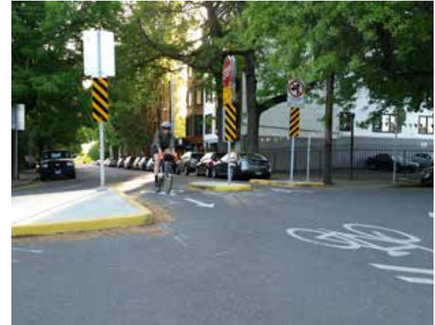
A neighborhood greenway with a traffic diverter. Source: Nelson\Nygaard
