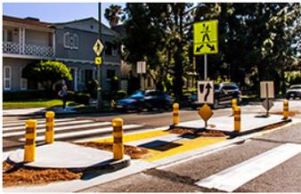
**Pedestrian Refuge Island** and medians create a safe space for pedestrians crossing the street, especially on streets with multiple travel lanes in one direction where speed tends to be higher.
