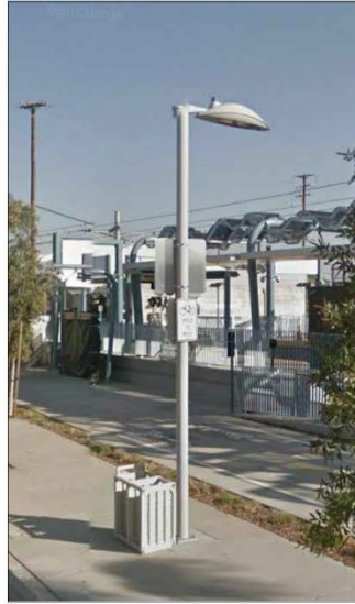
EXISTING PEDESTRIAN LIGHTING
