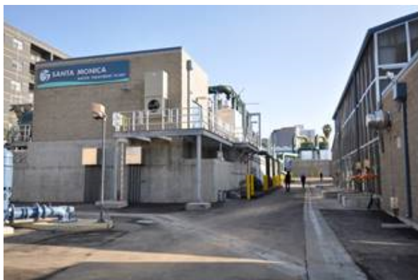
Incorporating the Latest Treatment Technologies Will Increase Production Efficiency to Greater than 90 Percent at the Arcadia WTP
