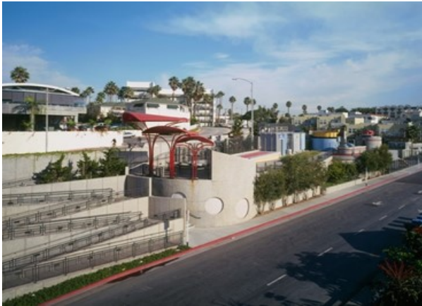
Existing SMURRF that will be Upgraded as Part of SWIP to Increase Recycled Water Production
