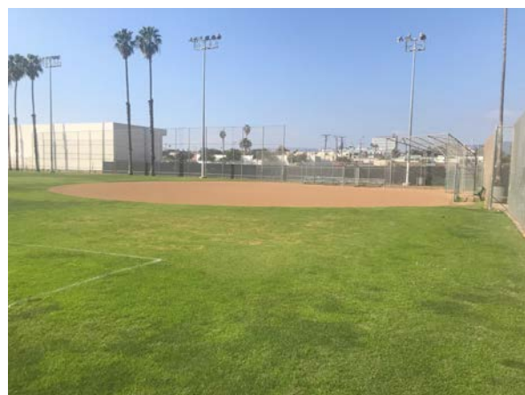
In addition to the existing buildings at Memorial Park, the baseball fields are characterized by backstops and tall fencing as well as stadium lighting.
