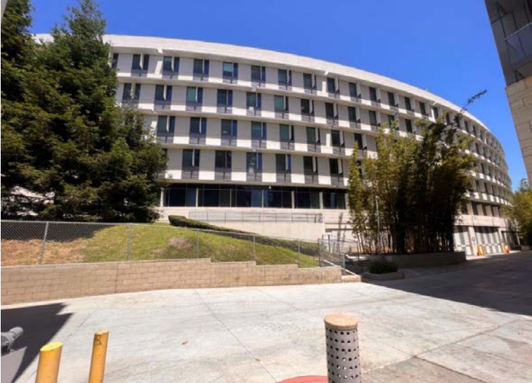
RAND Property/Existing Building - West/alley facade
