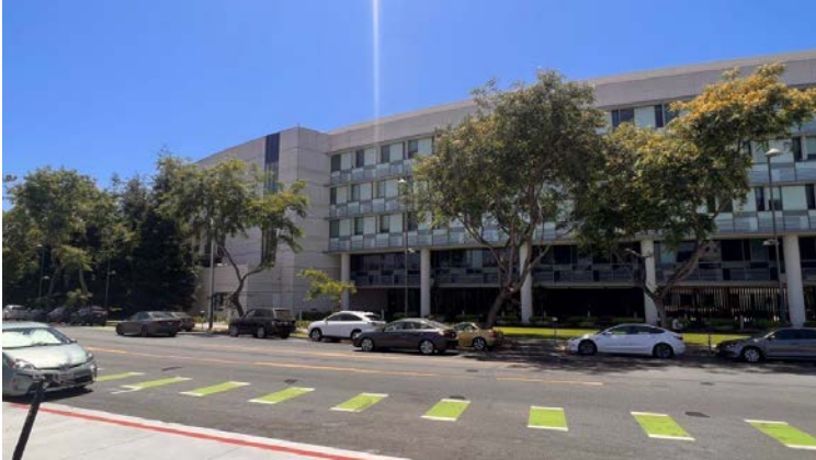
RAND Property/Existing Building - Main Street Frontage
