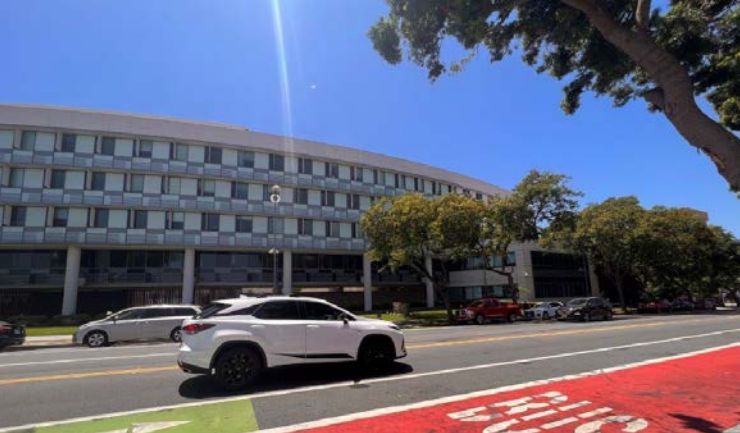
RAND Property/Existing Building - Main Street Frontage
