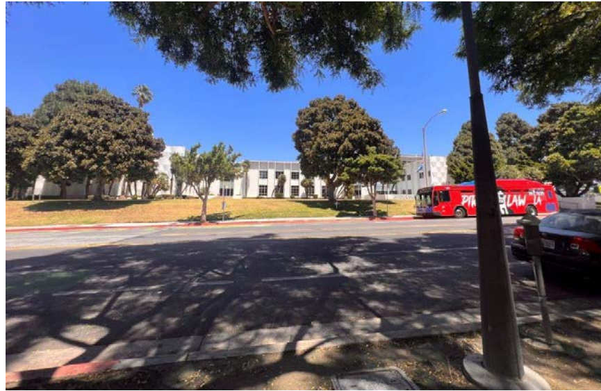
Courthouse building located across Main Street to the east of RAND
