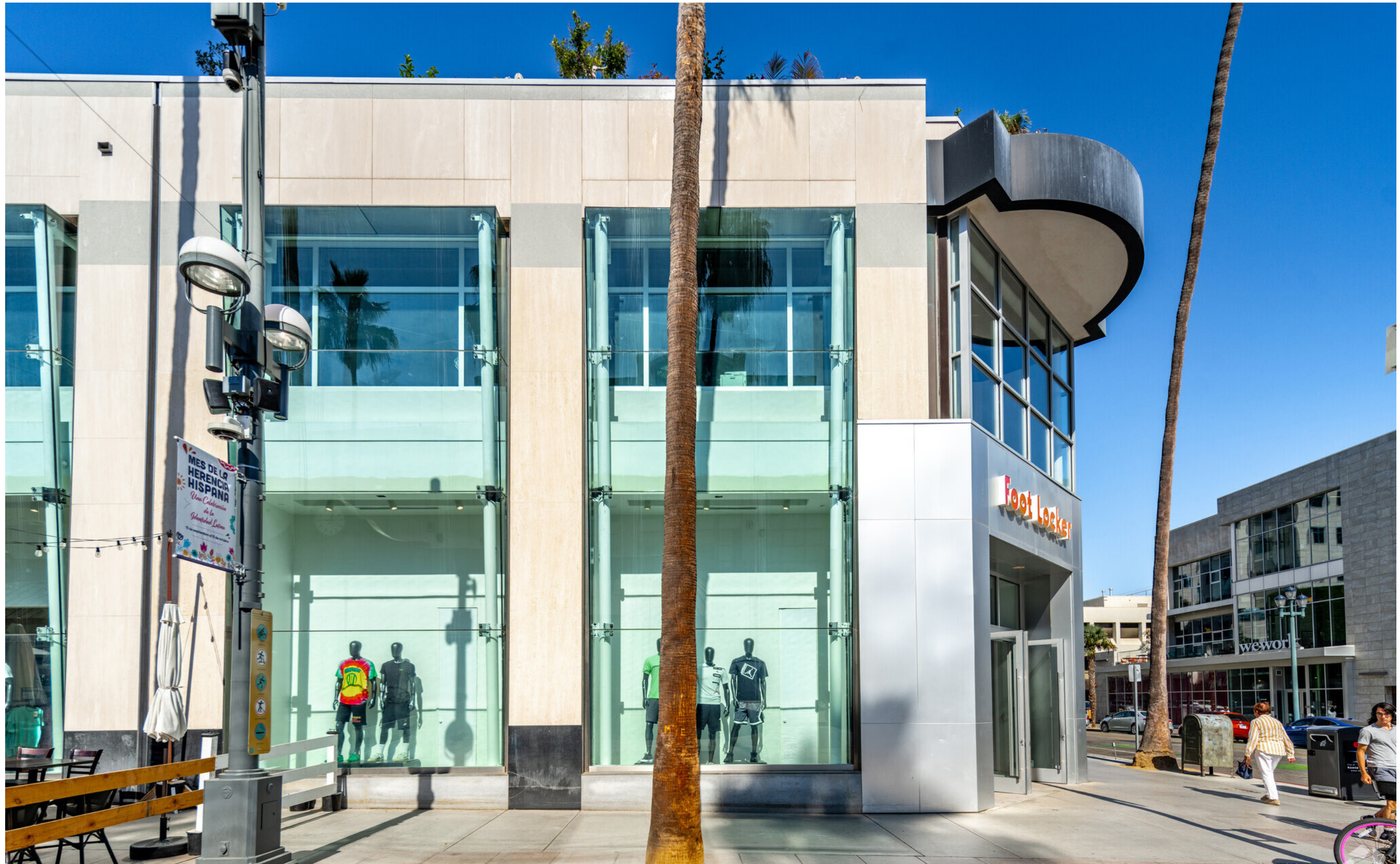
SITE PHOTOS 3RD STREET PROMENADE
