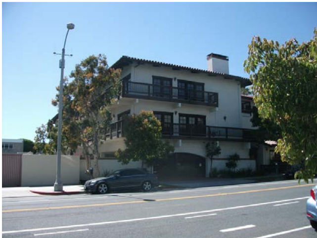
19. Northwest adjoining site
