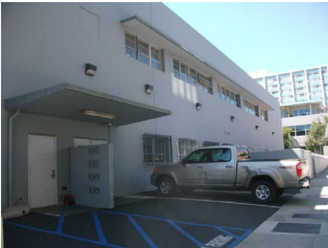
15. North adjoining site east facade
