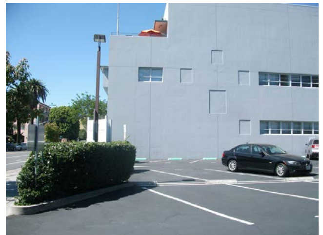
4. Southwest corner facing north
