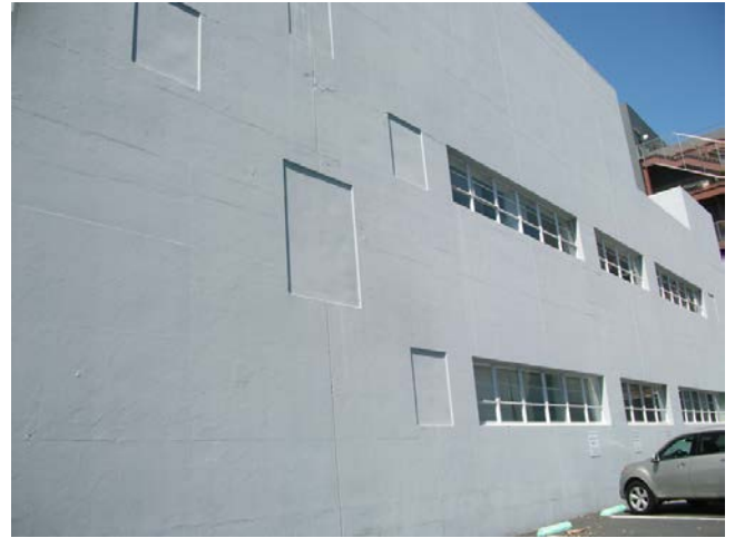
14. North adjoining site south facade
