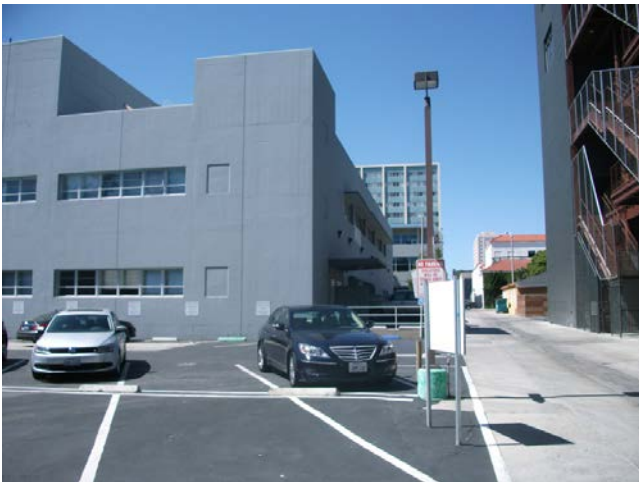
11. Southeast corner facing north
