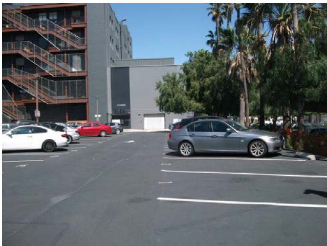
3. Southwest corner facing east
