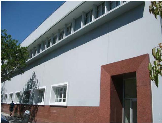
13. North adjoining site west facade
