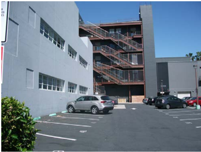
5. Northwest corner facing east
