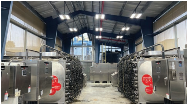
New Ultraviolet Light Advanced Oxidation Process added to remove industrial contaminants from the Olympic Well Field.
