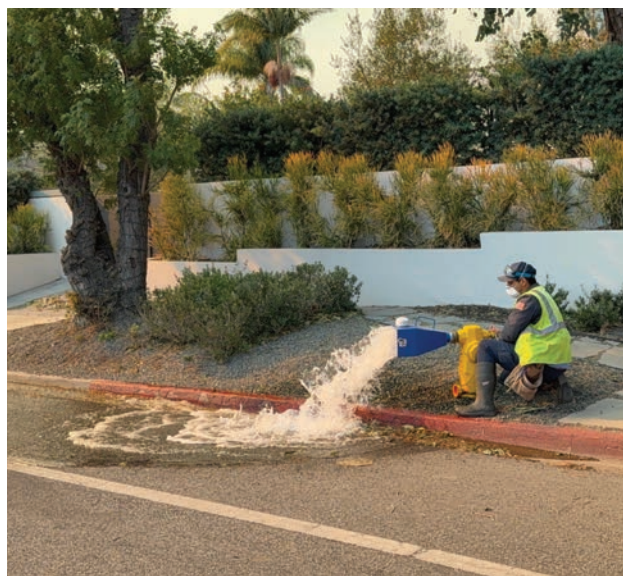
Operators Testing Fire Hydrants During the Wildfire Emergency to Ensure Operational Readiness.
