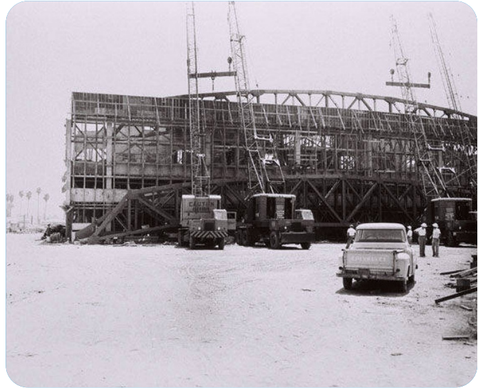
Construction of the Civic Center Auditorium in 1957 Source: Santa Monica Public Library
