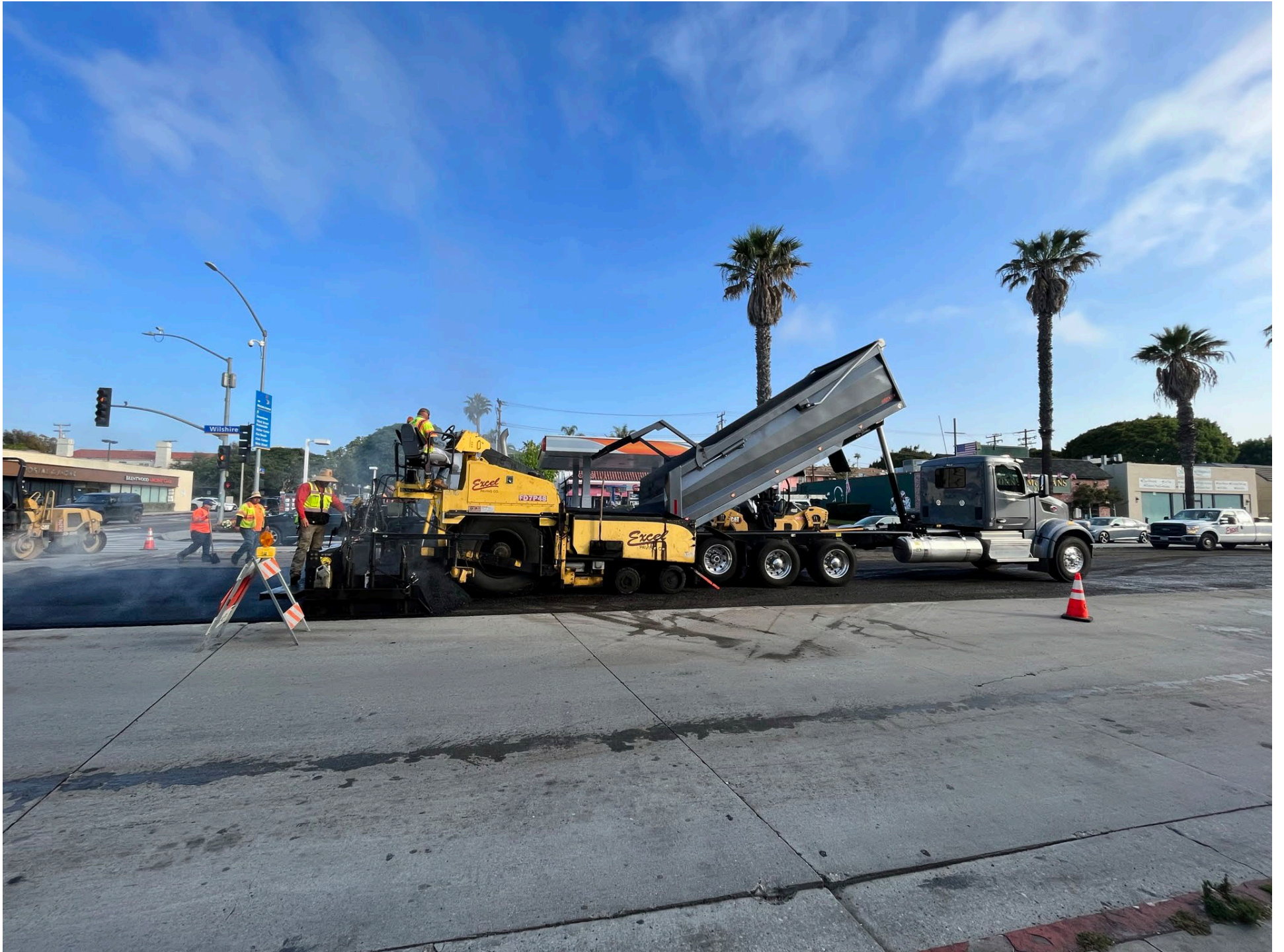
POURING ASPHALT ON WILSHIRE BOULEVARD + 26TH STREET
