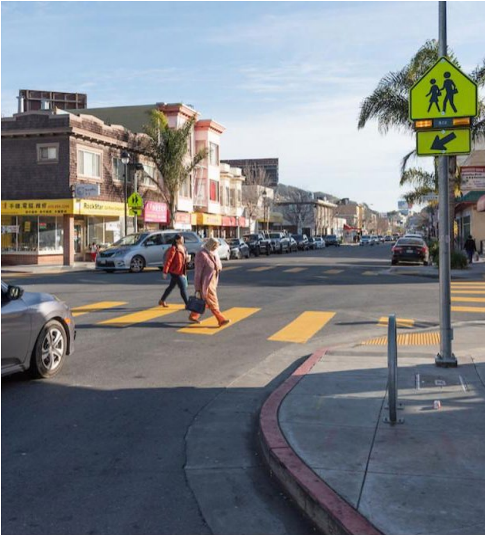
Flashing Crosswalk Beacon in San Francisco
