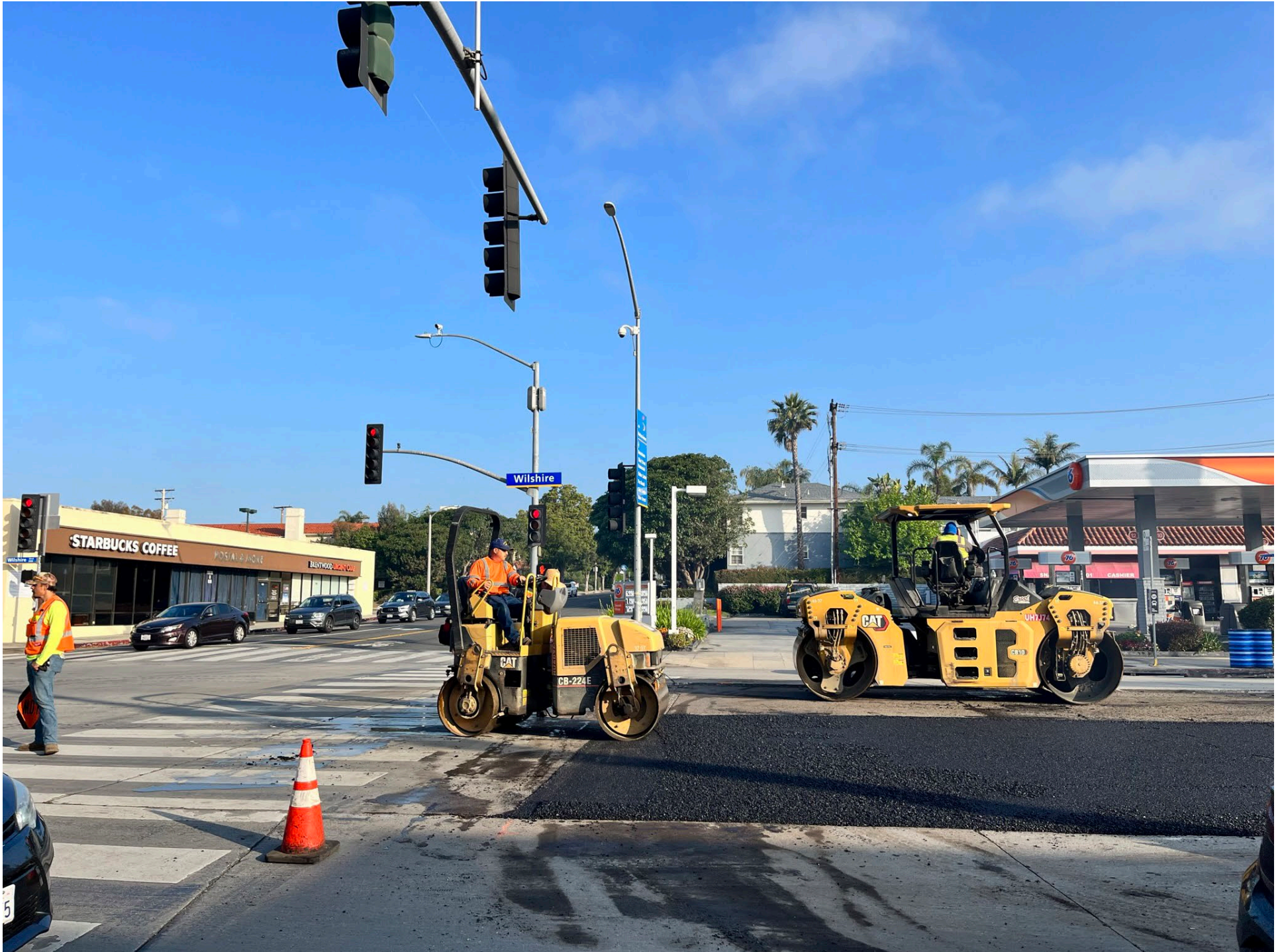
ROADWAY PAVING IN PROGRESS AT WILSHIRE BOULEVARD + 26TH STREET
