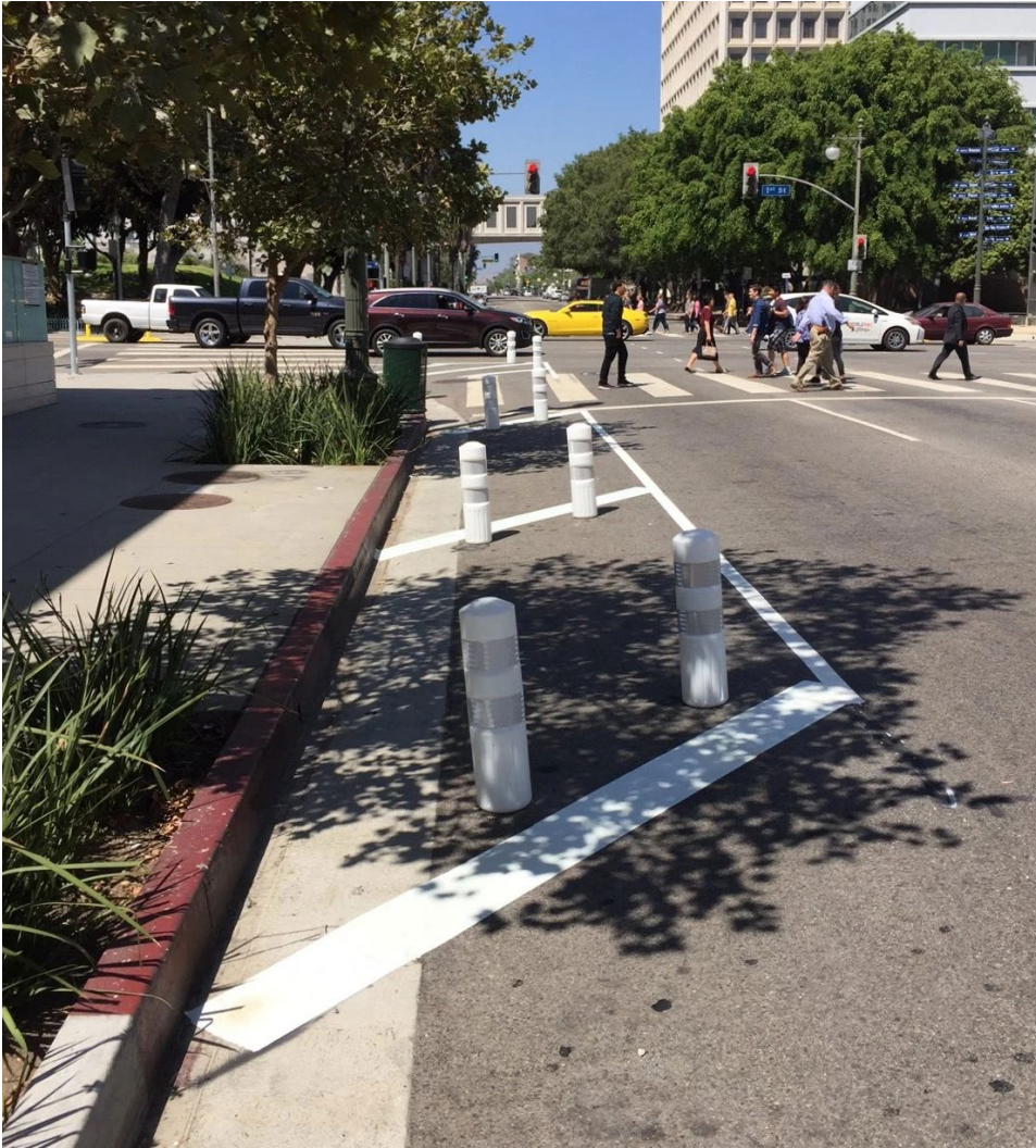
Paint and Post Curb Extension in Downtown Los Angeles
