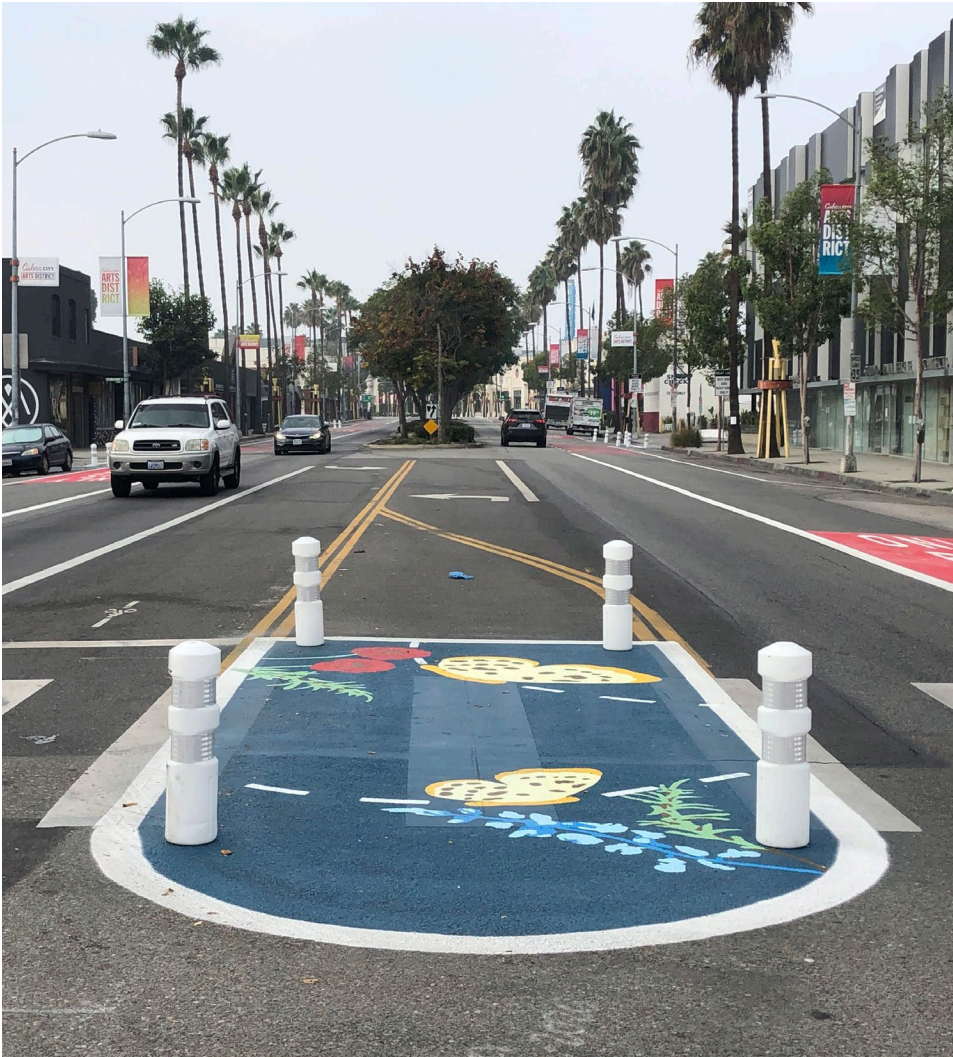
Pedestrian Median Refuge in Culver City
