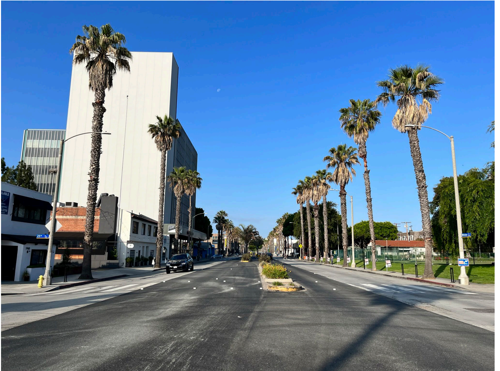
FRESH ASPHALT AND TEMPORARY ROADWAY MARKERS DURING CONSTRUCTION AT WILSHIRE BOULEVARD + 25TH STREET
