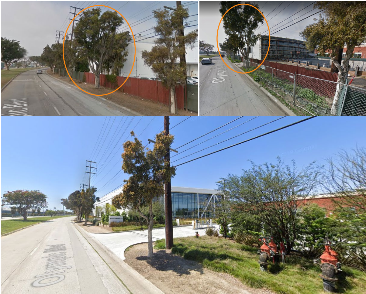
Restitution resolved, posted and removed for Fire & vehicular access at the "Pen Factory" remodel 2701 Olympic Blvd.
